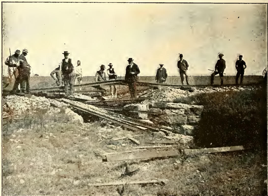
Culvert blown up by the Boers, Chieveley. Mended the day before the battle of Colenso
