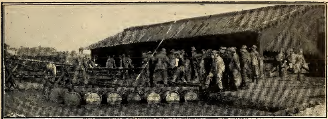
Making a barrel pontoon
