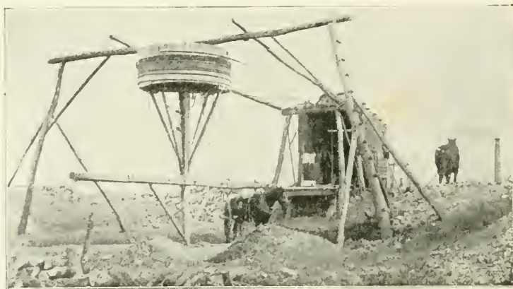
THE INFANCY OF A GOLD-MINE: WINDING QUARTZ WITH A WHIM
