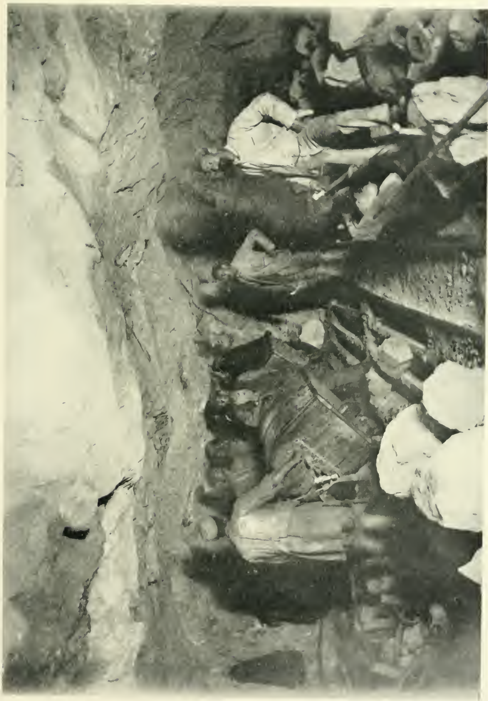
DRIVING AN "END" IN MAY CONSOLIDATED MINE, JOHANNESBURG
